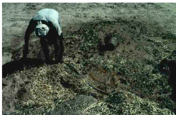
Figure 9. Mixing mud with straw and water
