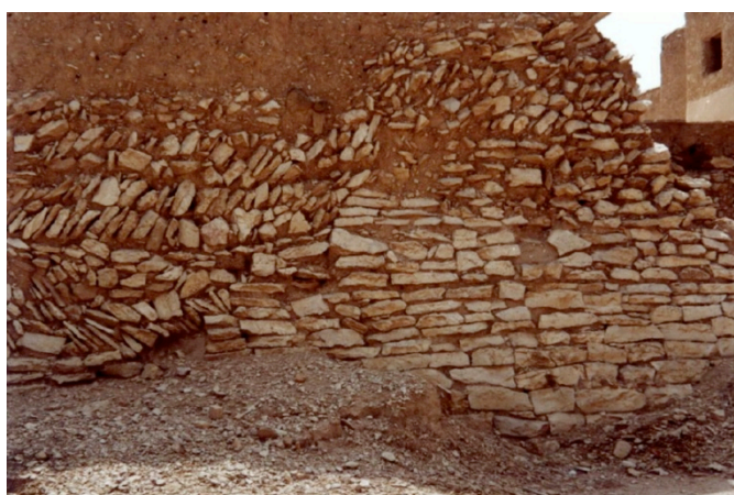
Figure 12. Stones of the lower part of an adobe wall, al-Dar'iyyah, Najd
