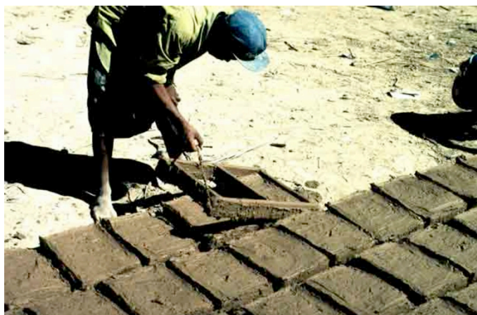
Figure 10. Pressing adobe mixture into wooden frames
