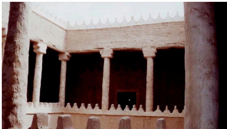
Figure 7. Crenellated parapets redirect raindrops away from the mud walls
