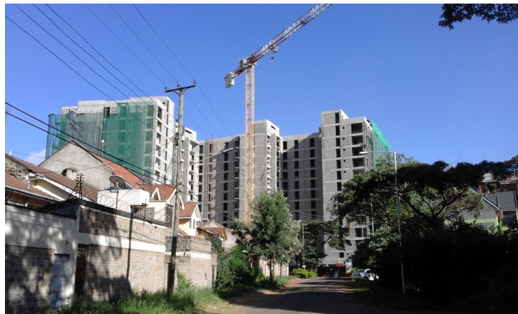
Figure 3. New high-rise multi-unit apartment blocks in Kileleshwa , Nairobi. author, 2015.
