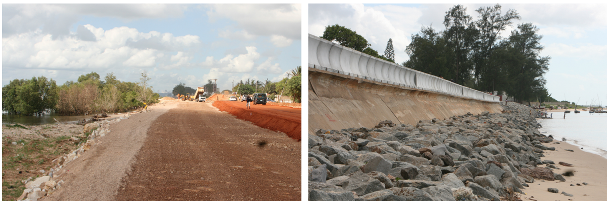
Figure 7. Mangrove destruction for the ring road construction; flood retention wall at Bairro dos Pescadores (2015)
