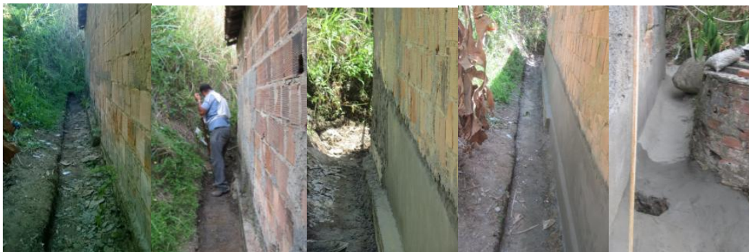
Figure 3. Waterproofing works in the back a house involved in the Architect of the Family project (before, during and after the works)
