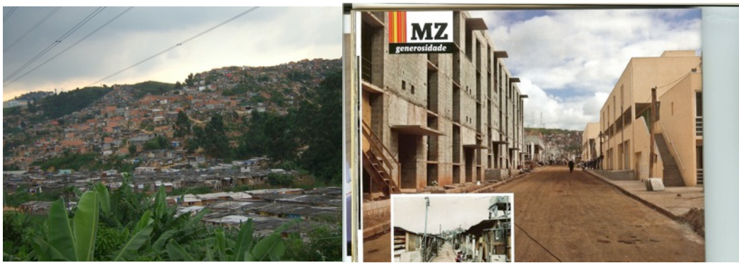
Figure 1. The community of Portais do Campo before (in the original favela) and after the resettlement process (during the construction of the new affordable houses)
