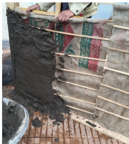
Figure 4. First Panel, Figue's tissue with earthen cement mixture
