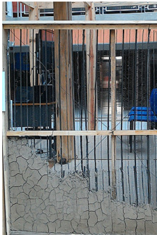
Figure 8. Third Panel, steel mesh core with two earthen mixtures layers.
