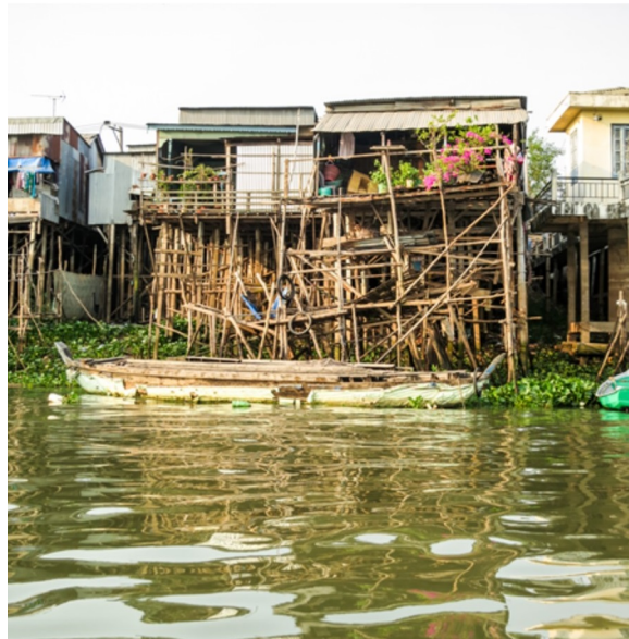
Figure 3. Chau Doc traditional house built in the margins of the Bassac River.
