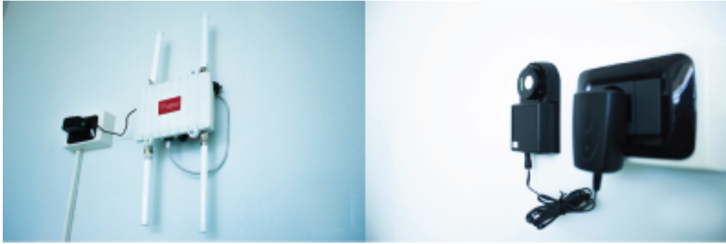
Figure 5. Crowd-sensor (left) and temperature, humidity and CO 2 sensor (right) installed in the out-loud study room at CLE.
