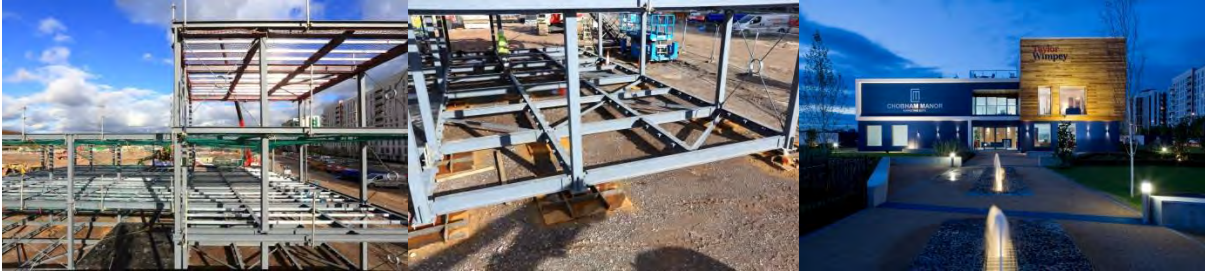
Figure 2: Chobham Manor, the steel frame, foundation pad, and finished buildings, photo credit: Rob Brown Photography
