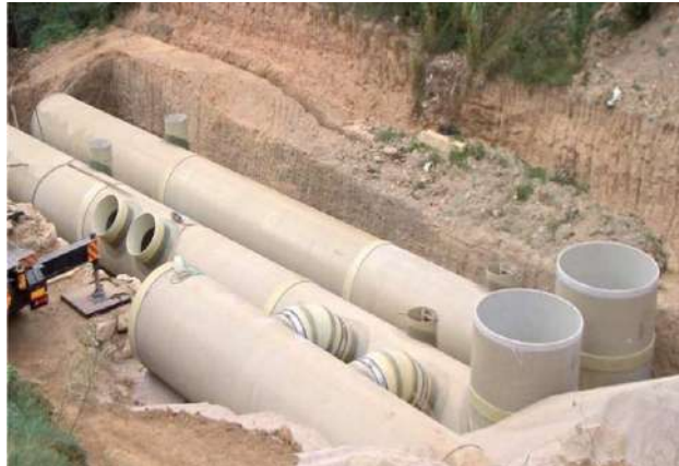
b) GRP Tanks (Taken from AMITECH, 2010).
