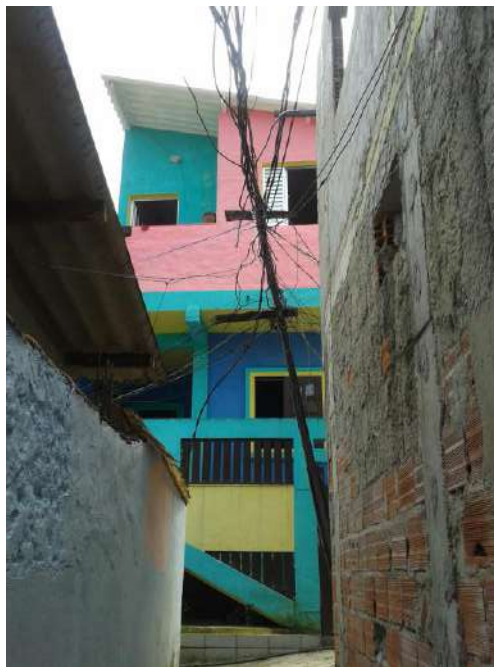
Figure 6. Popular solution to remedy the lack of electric system in Vila Sahy. Note. Photograph taken by the author, 2015.
