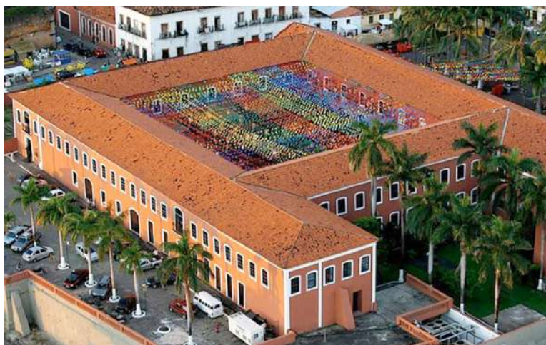
Figure 2. Aerial view of the Convento das Mercês, construction of 1654, in the image decorated for the feasts of the saints in the month of June (Source: Kartagener2, Flickr, 2013).
